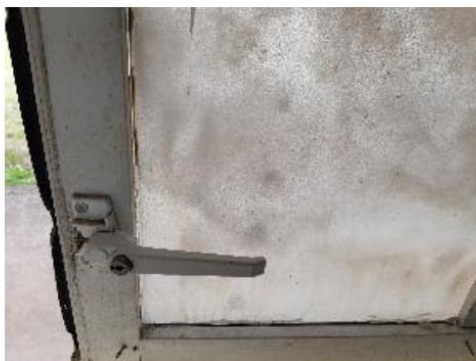
11 Ease and adjust all windows and replace faulty hinges and handles. Remove nails
