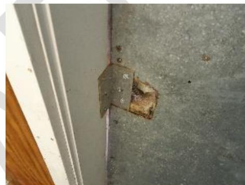
12 Exit door at the kitchen has been 'modified/sealed' in poor condition
