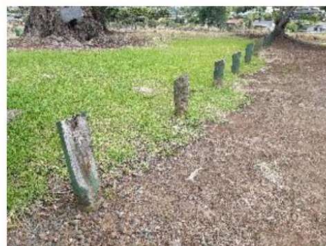
2 To replace damaged timber bollards
