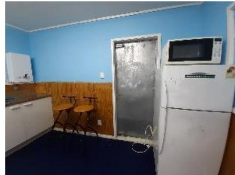
4 Exit door in poor condition – currently not openable and 'sealed' for security
