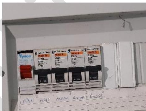
10 Power supply for the building – 60A
