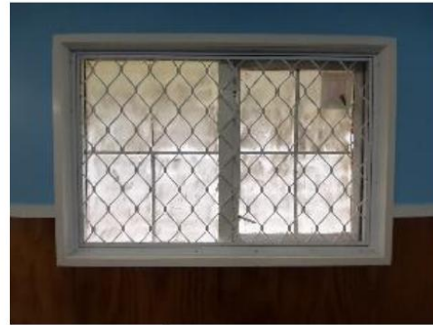
10 Window with metal grills and Perspex lining has been installed
