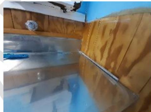
6 Rubber 'sealant' for steel sink to be remediated
