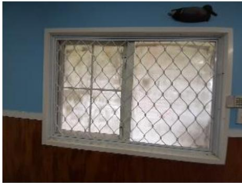
9 Window with metal grills and Perspex lining has been installed for security
