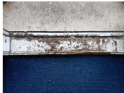
14 Threshold for main door entrance with wear and tear
