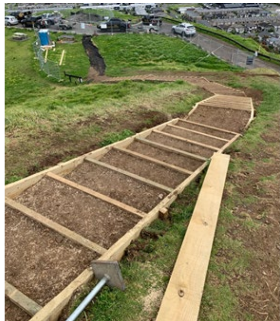
Photo 4: Maungarei boxed step replacement progress
